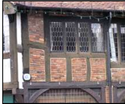
Close up of Angel Buildings
