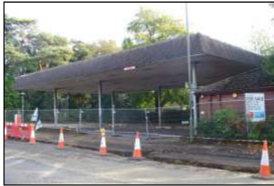
Derelict garage site at on old A3 spur to the north
