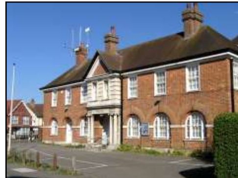
Former Police Station
