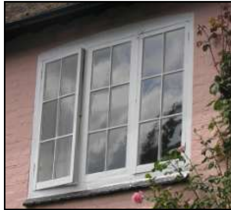
Wooden window frame, Courts Mount Road
