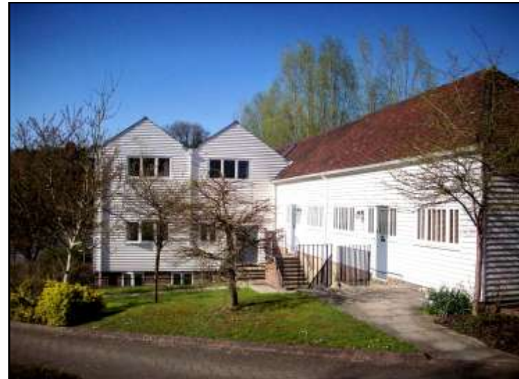
Sickle Mill, restored
