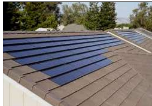
Examples of integrated solar photovoltaic panels
