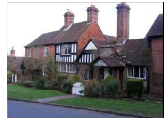
Petworth Road, Courts
